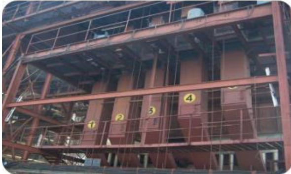
Bagasse Silos & Feeders of Boiler
